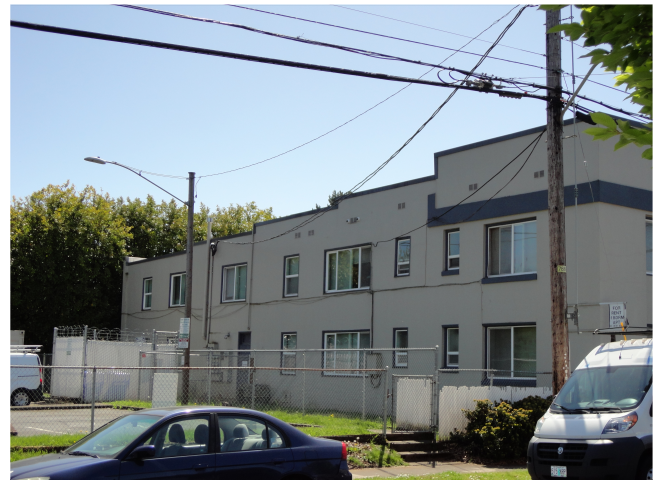
Exterior Parking Lot View
